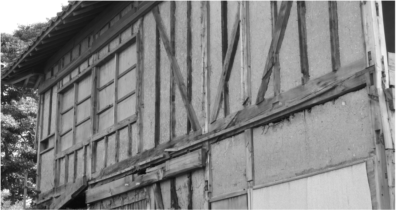
4) Aikawa. Traditional house realized with wood and earth, a construction method still in use (O.N. 2014).
